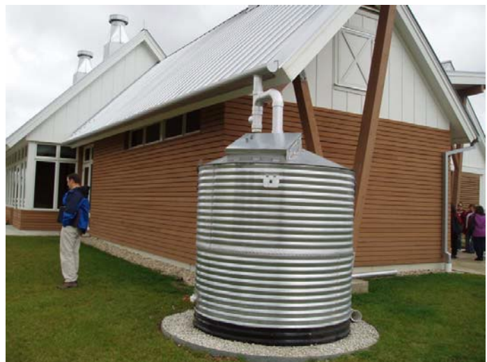
Figure 3.3b: Above Grade Cistern
