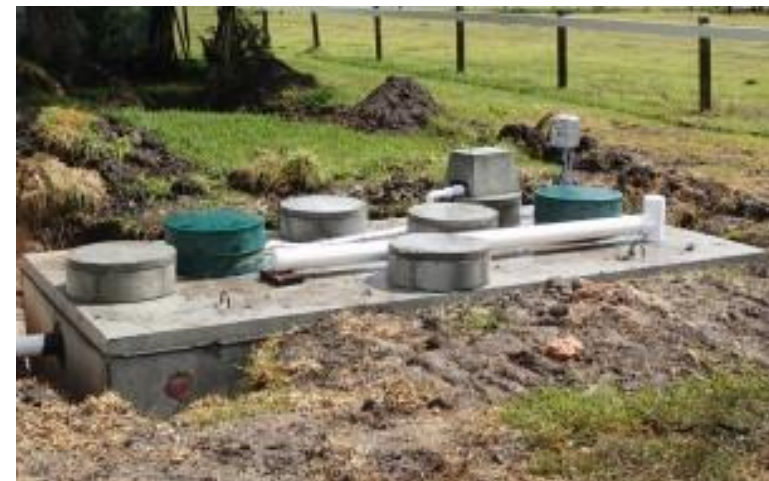
ATU with built-in Trash Trap
